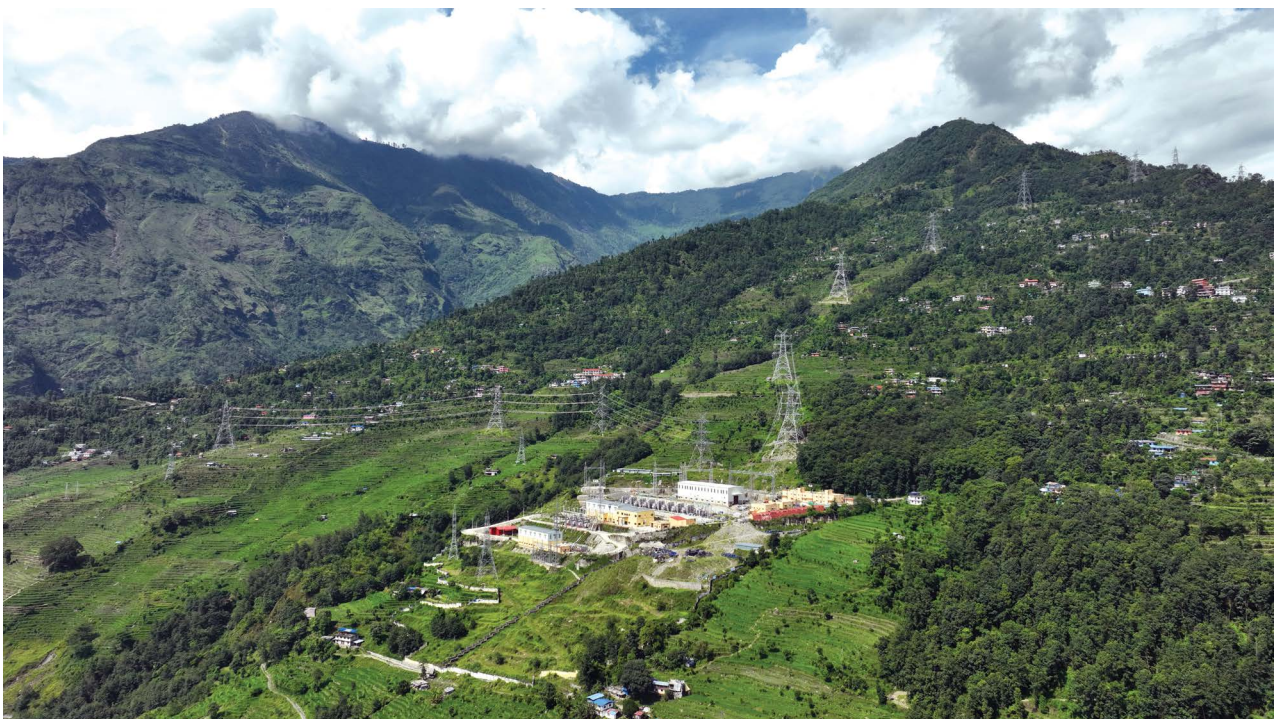
Barhabise 400/220/132 KV Substation Under Construction.
