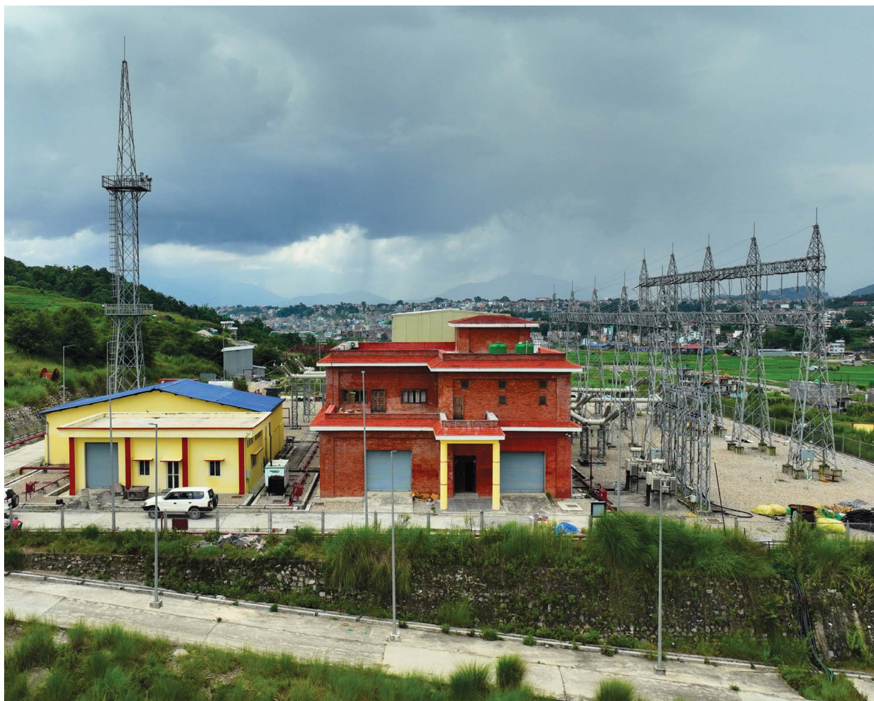
A view of the 132/11 KV Changunarayan Substation Infrastructure and Control Buildings.
