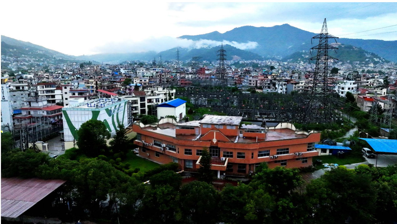
Load Dispatch Centre, Siuchatar
