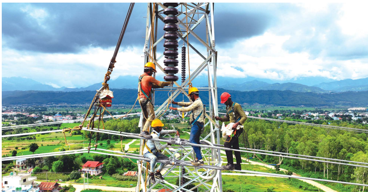
Conductor Stringing Work in Progress for the 400 KV Dhalkebar-Hetauda Transmission Line in Hetauda
