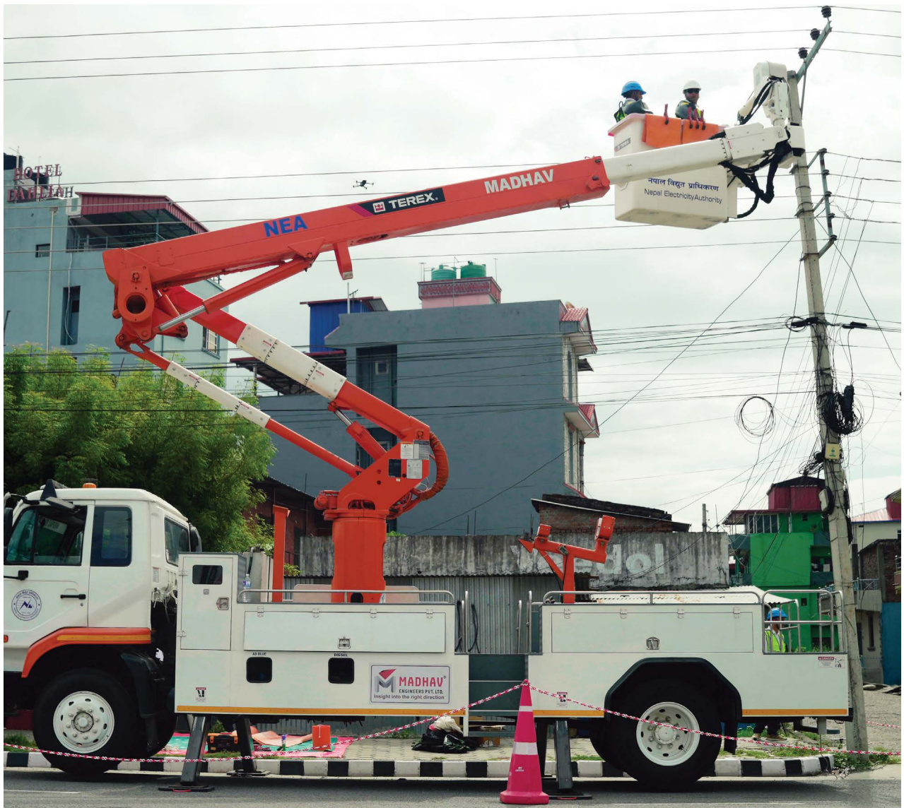
Liveline Maintenance in Action: NEA Technicians Working Safely to Ensure Uninterrupted Power Supply in Butwal.
