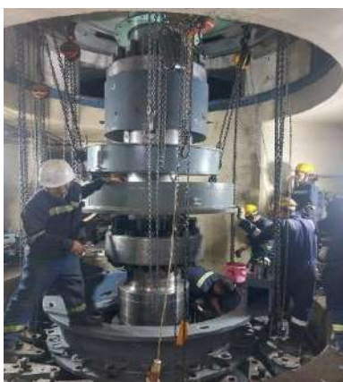
Overhauling of Unit No 2
