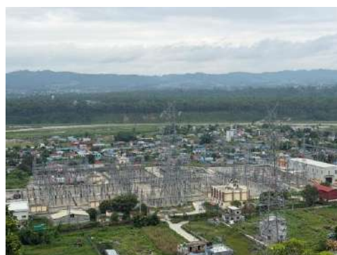
400/220/132/11 kV Hetauda Substation
