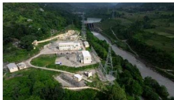
Udipur Substation in Lamjung District
