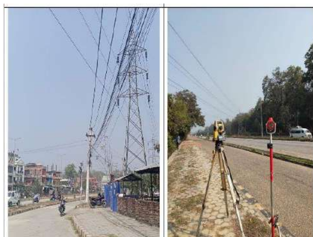
Check survey of the existing 66 kV double-circuit line
