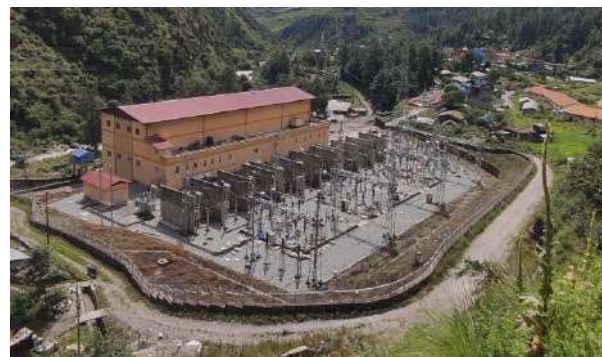
Powerhouse and Switchyard of Sanjen Hydropower Station
