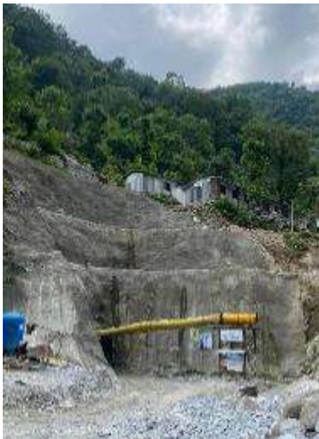
HRT Inlet Portal
