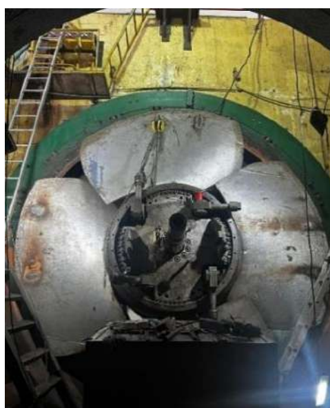
Kaplan Runner during Overhauling of Unit No2
