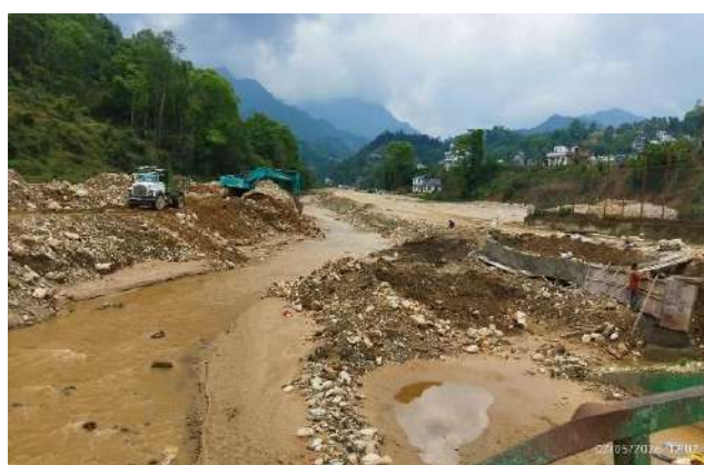
Construction of Retaining Plum wall at Intake Site
