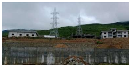
Pangtang Substation Under Construction
