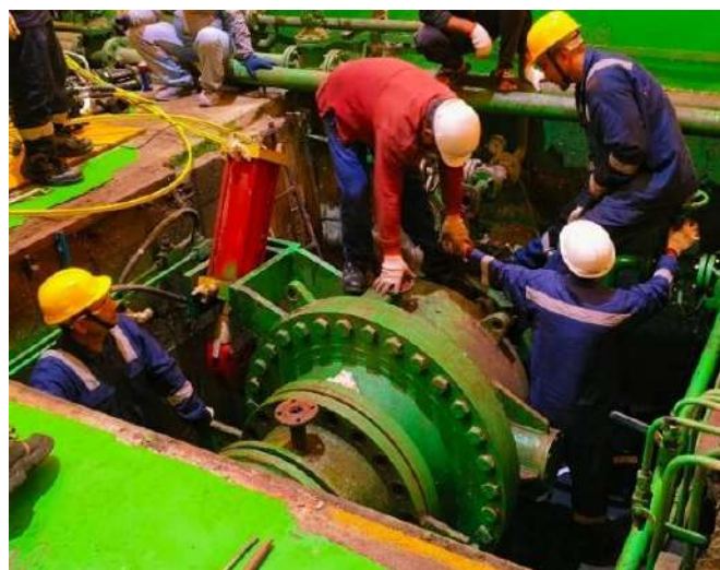
Dismantling of MIV
