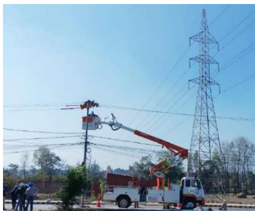
Live Line Maintenance work under Bhaktapur DC
