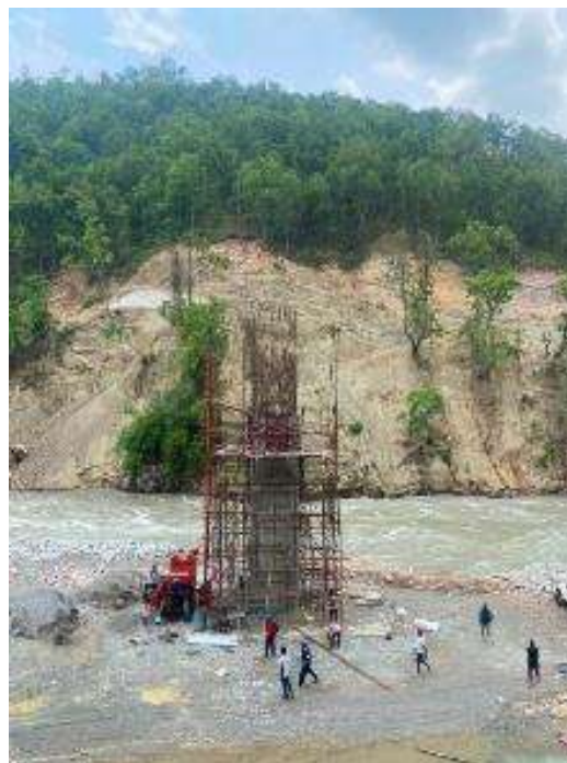
Construction of Motorable Bailey Bridge at Dudhkoshi River About
