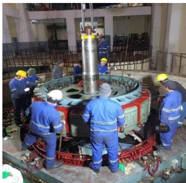
Installation of Rotor Pole of Unit No 2
