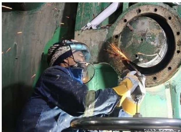
Repair of Main Inlet Valve
