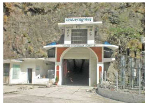
Chilime Hydro Power Plant
