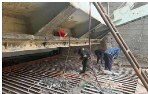
Radial Gate Maintenance
