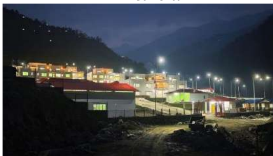
Camp Facilities at Syauli Bazar, Kaski
