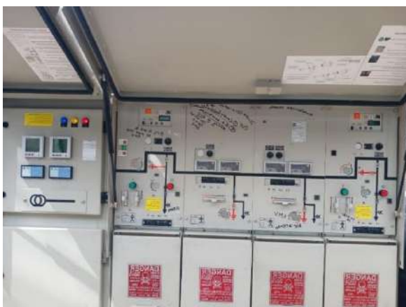
Charging of 11 kV RMU for Bhaktapur-FDR-A
