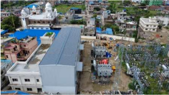
132/66kV GIS Substation Extension
