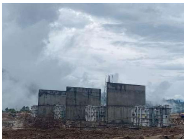
Transformer Foundation at Lapsipedi Substation
