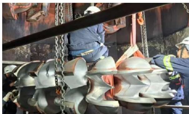
Overhauling of Unit No 2
