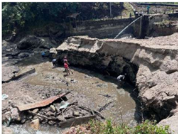
Debris Cleaning at Intake Site
