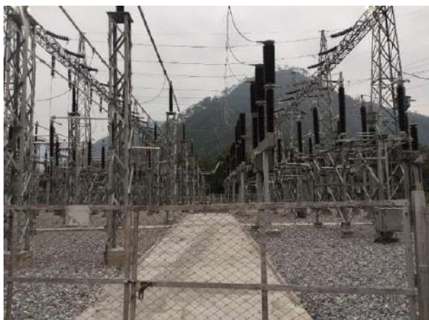
Completion of two 132 kV bay expansion works at New Modi Substation
