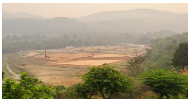
Damauli substation Piling works
