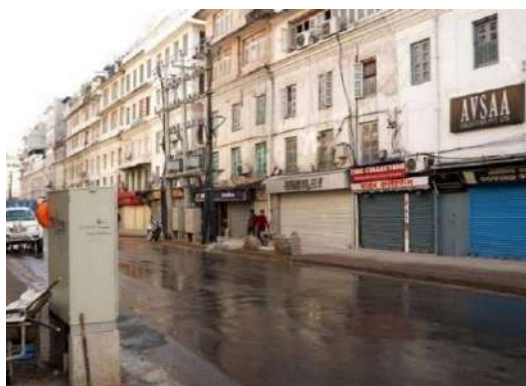
Indrachowk Area after dismantling of poles
