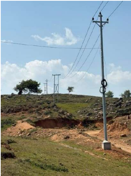
Construction works of 33 kV Line
