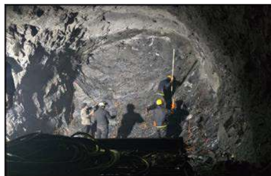
Explosive Loading at Tailrace Tunnel of RKHEP
