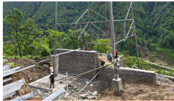
Transmission Line Tower Erection Work
