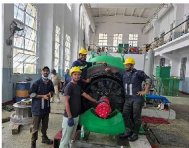
Overhauling of Unit No 2
