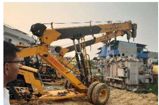
Shifting Power Transformer
