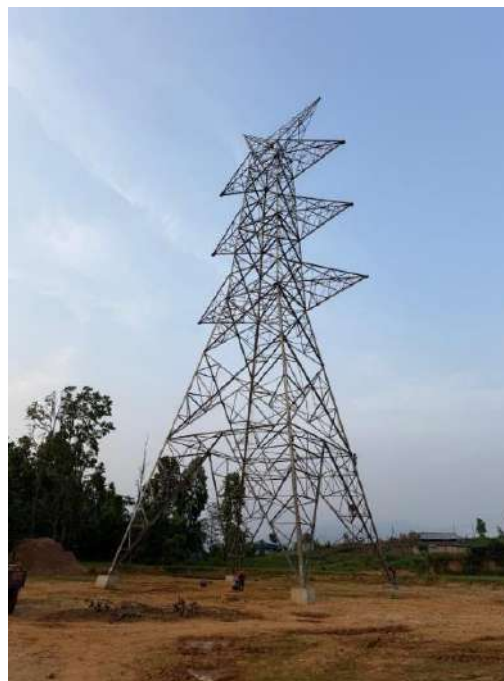
400 kV erected tower
