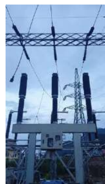
T.C.B. 132 kV breaker installation
