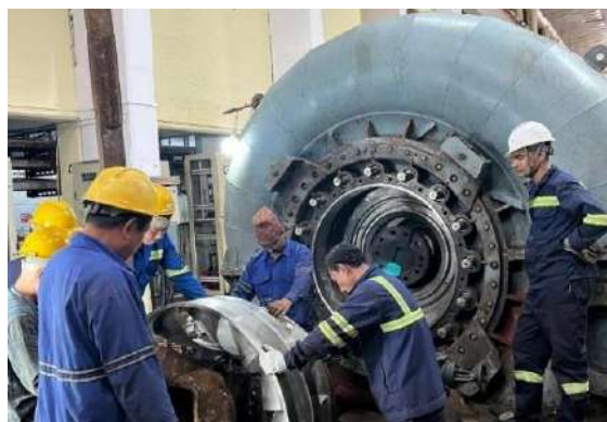
Overhauling of Unit No 6
