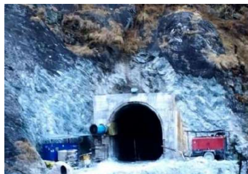
Adit 3 under construction
