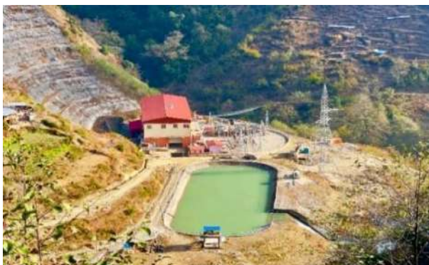
Powerhouse Area of Sanjen (Upper) Hydropower Station
