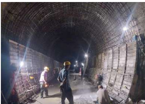
Construction Activities in Headrace Tunnel
