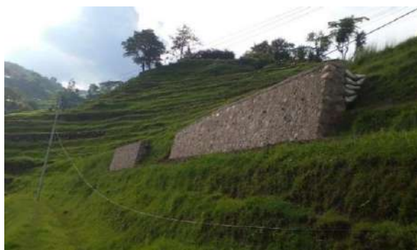
Construction of Retaining Wall
