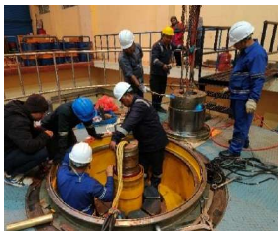
Replacement of Thrust Collar
