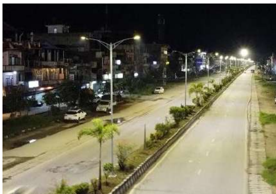
Smart Street Lights in Ratnapark
