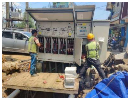
RMU Installation work in Pokhara
