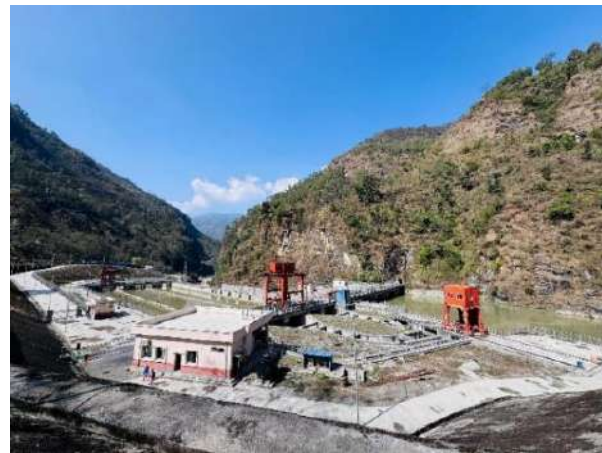
Panoramic view of the completed headworks, intake structures, and desander basin at the Chaku site in Sindhupalchok
