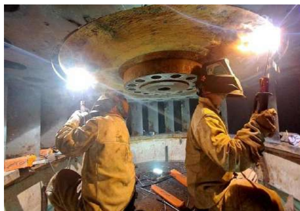
Maintenance of Turbine Headcover
