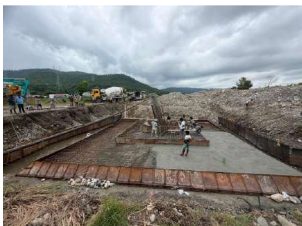
400 kV multi-circuit tower foundation
