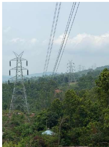
400 kV double-circuit Quad ACSR Moose conductor stringing in the Makwanpur forest area
