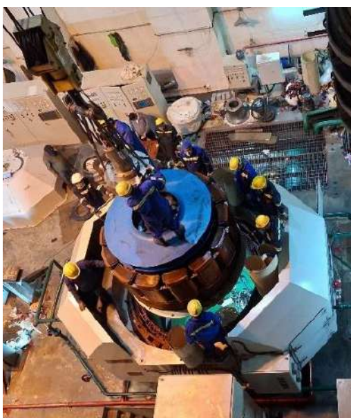
Assembly of Generator Shaft and rotor of Unit 1
