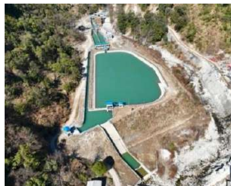
Headworks Area of Sanjen (Upper) Hydropower Station
