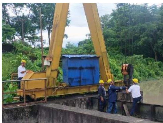
Intake site Gearbox Maintenance
