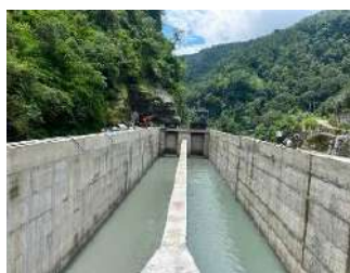
Maintaining Desander Level for various wet tests
