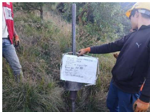
Soil investigation at a transmission-line tower location
