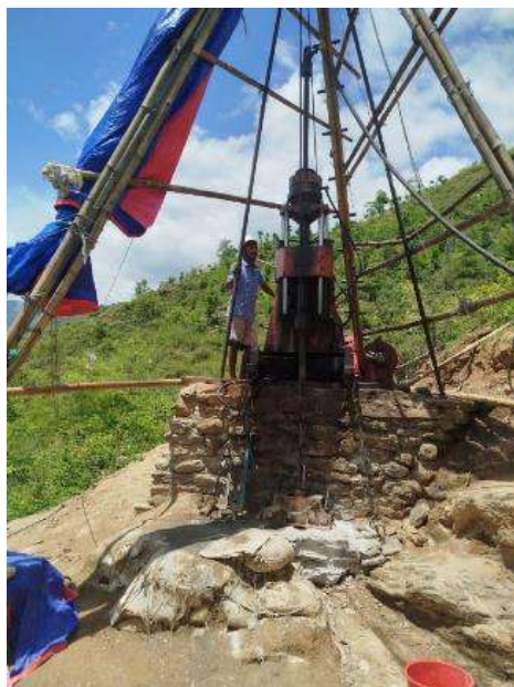
Bore Hole Drilling at Main Powerhouse Area
