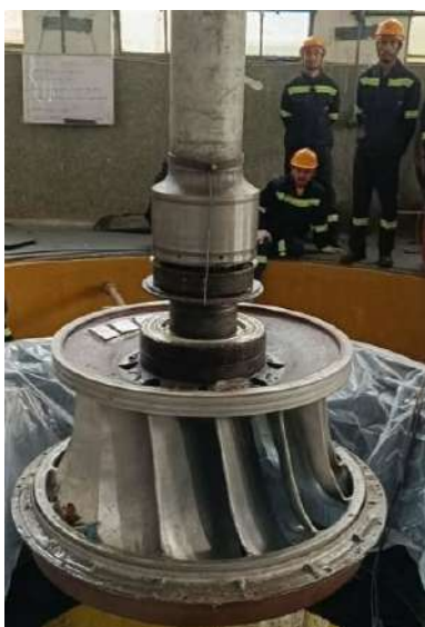
Overhauling of Unit of 1
