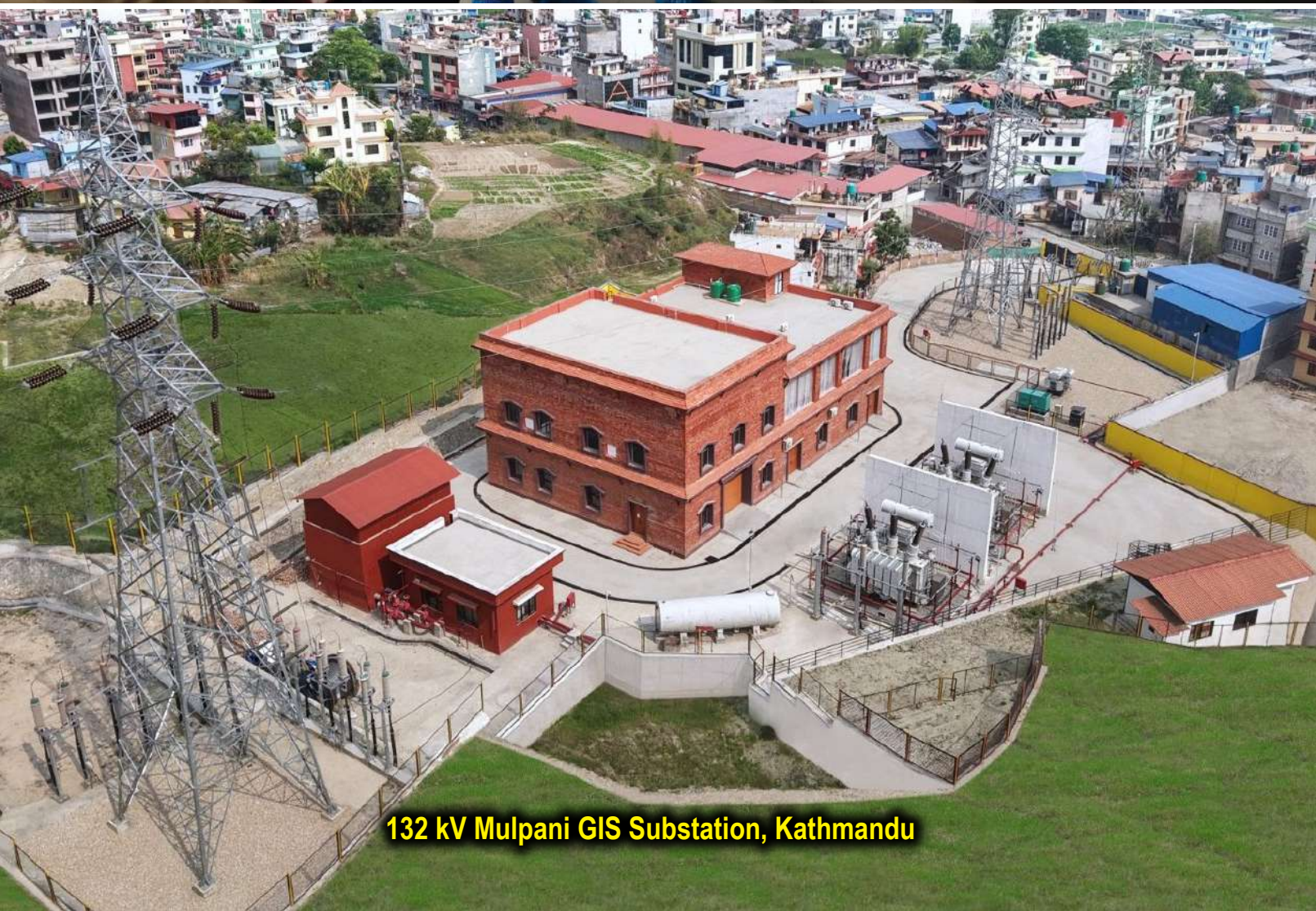
Joint Inauguration of Markichowk and Mulpani Substation from LDC by ADB President, Hon'ble Minister and Norwegian Ambassador
