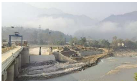
Right Bank Protection Works
