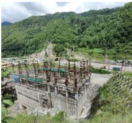
Overview of Powerhouse
