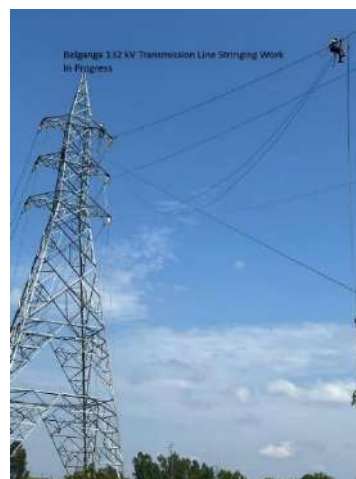
Balganga 132 kV transmission-line stringing work
