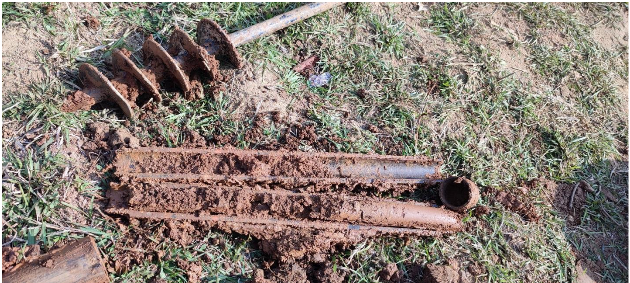
Soil Sample in Split Spoon Sampler of Transmission Tower BH 3
