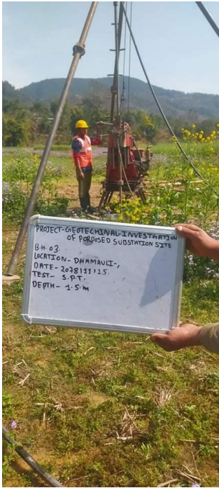
Conduction of Standard Penetration Test at New Borehole 3 of Damauli SS; Depth 7.5 m
