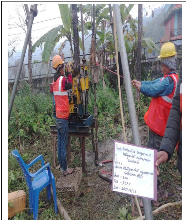
Conduction of Dynamic Cone Penetration Test at Depth 3.0 m
