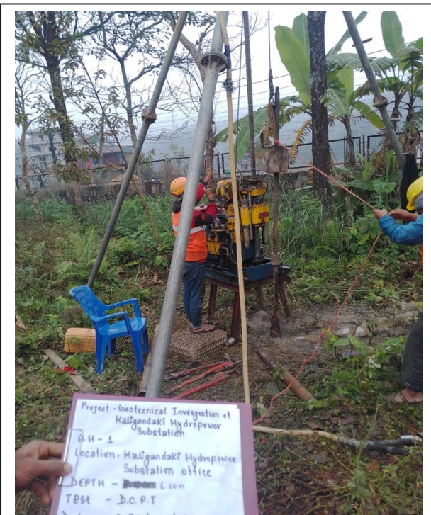
Conduction of Dynamic Cone Penetration Test at Depth 6.0 m
