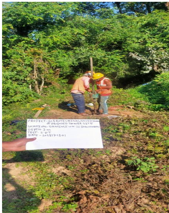
Conduction of Standard Penetration Test at Depth 3.0 m
