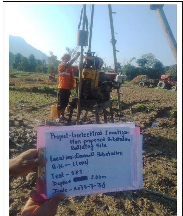
Conduction of Standard Penetration Test at Depth 9.0 m
