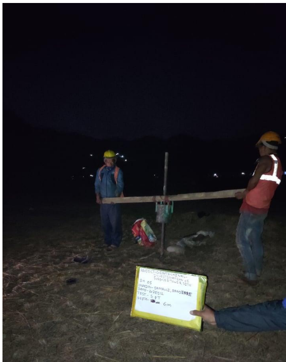
Conduction of Standard Penetration Test at Depth 6.0 m
