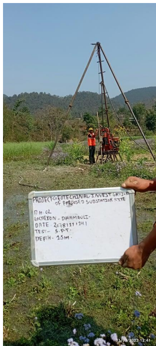
Conduction of Standard Penetration Test at New Borehole 2 of Damauli SS; Depth 1.5 m
