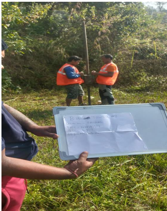
Conduction of Standard Penetration Test at Depth 1.5m
