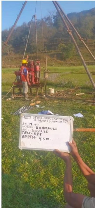
Conduction of Standard Penetration Test at New Borehole 1 of Damauli SS; Depth 4.5 m
