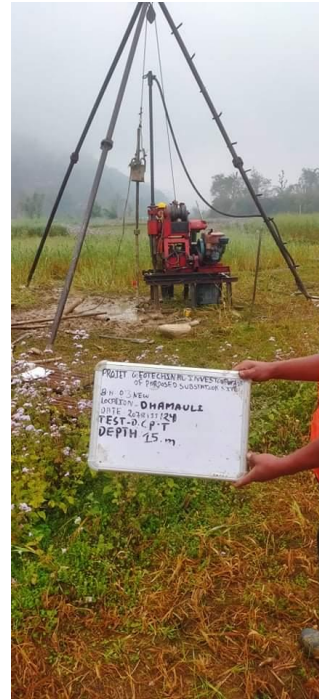
Conduction of Dynamic Cone Penetration Test at New Borehole 3 of Damauli SS; Depth 15 m
