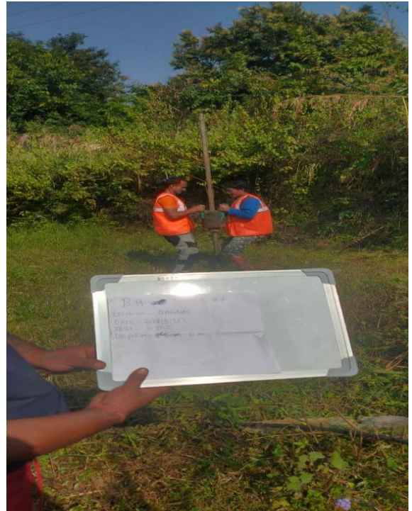
Conduction of Standard Penetration Test at Depth 6.0 m
