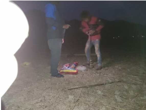
Drilling by Auger
