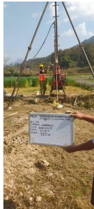
Conduction of Dynamic Cone Penetration Test at New Borehole 4 of Damauli SS; Depth 13.5 m
