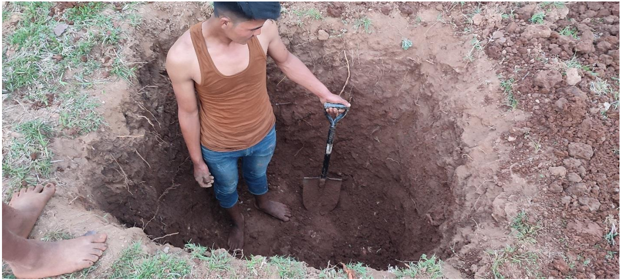
Excavation of Trial Pits in Transmission Tower Location BH 3
