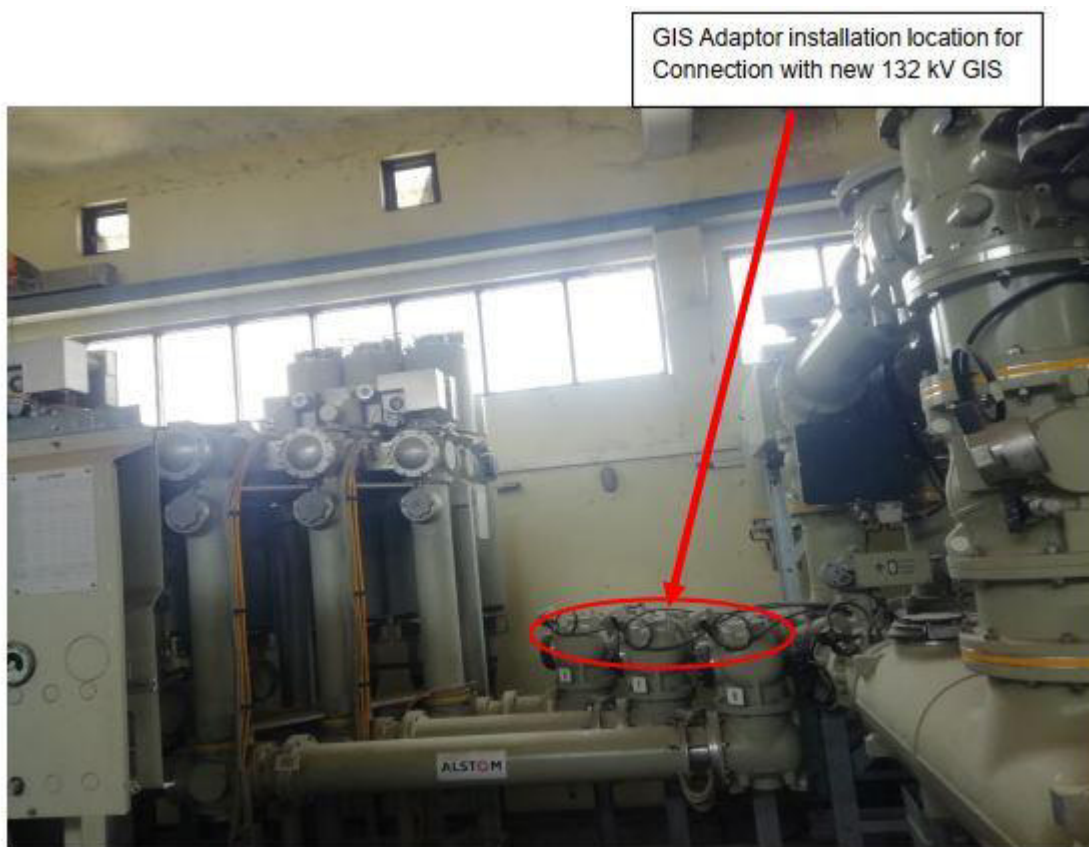
Figure 1 : GIS Adaptor at Existing 132 kV GIS
