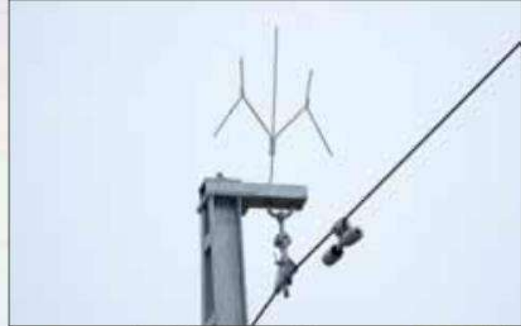
Wishbone Prevents Bird Landing on Wire
