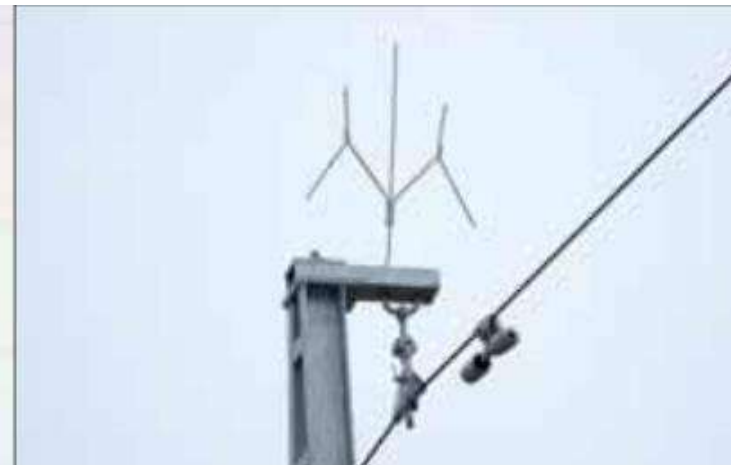
Wishbone Prevents Bird Landing on Wire
