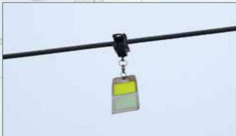
Bird Diverting Reflector
